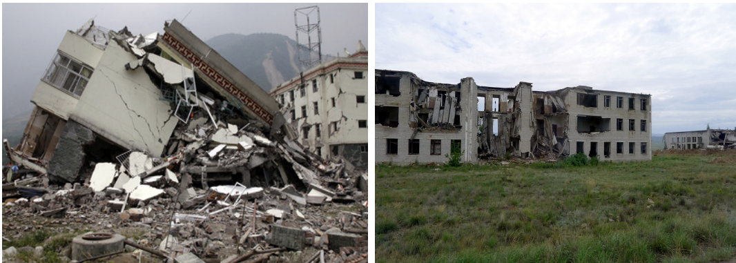
Figure 1. Collapsed[19] and Dilapidated Buildings[20]
