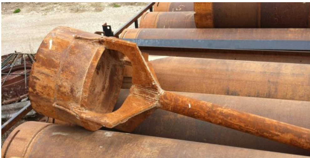
Figure 1.3 Upsizing Reamer to Fit 25.5-Inch OD Casings, Casings in Background
