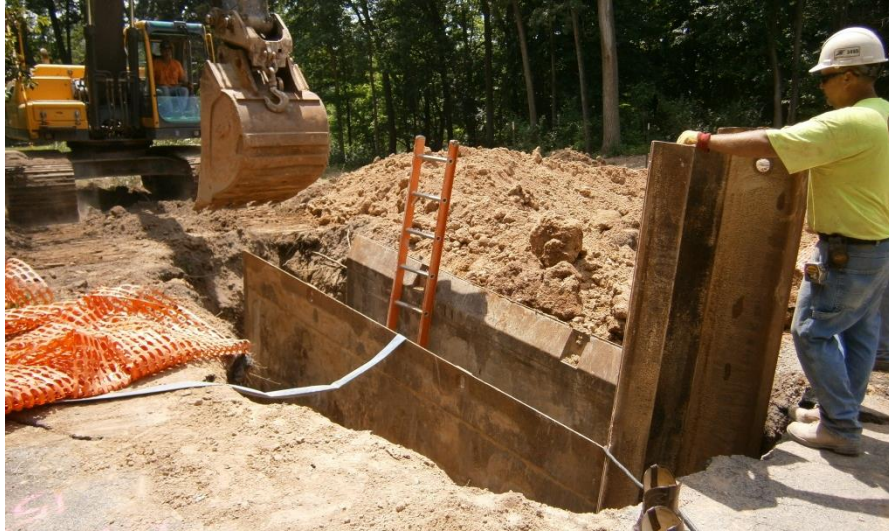
Figure 3.1 Exit Pit Installation for PT/HDD Procedure
