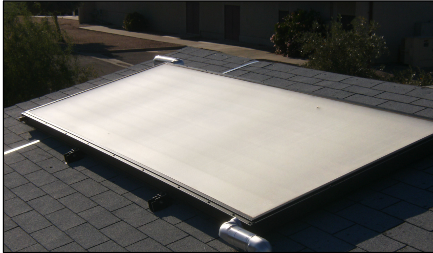
Figure 10. SunEarth® Flat-Plate Collector
