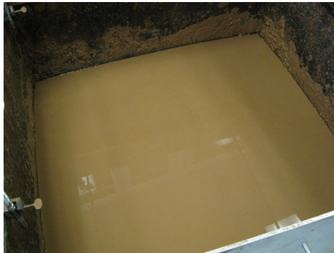
Figure 3.8 Preparation of Soil Bed
