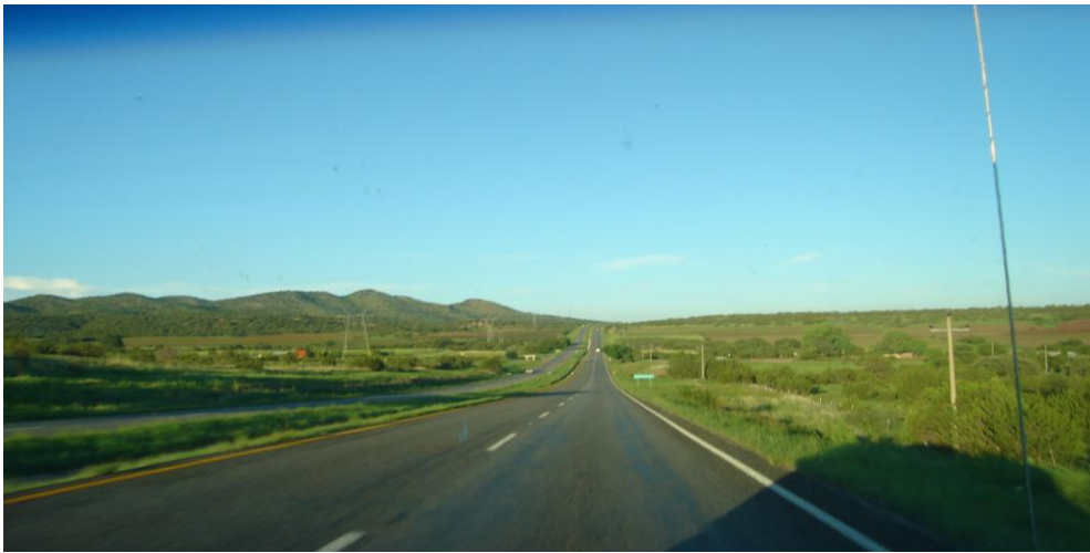
Figure 16 Road to the city of Cuauhtémoc. (Photo Jesus Estrada)
