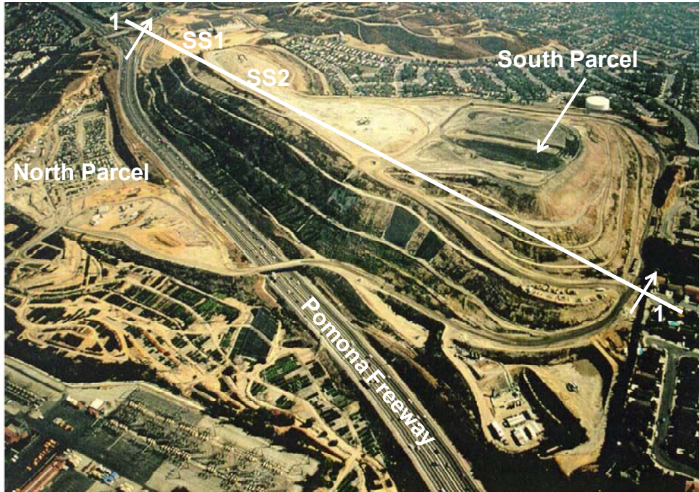
Figure 10-1 Aerial View of OII Landfill (Matasovic and Kavazanjian 1998)
