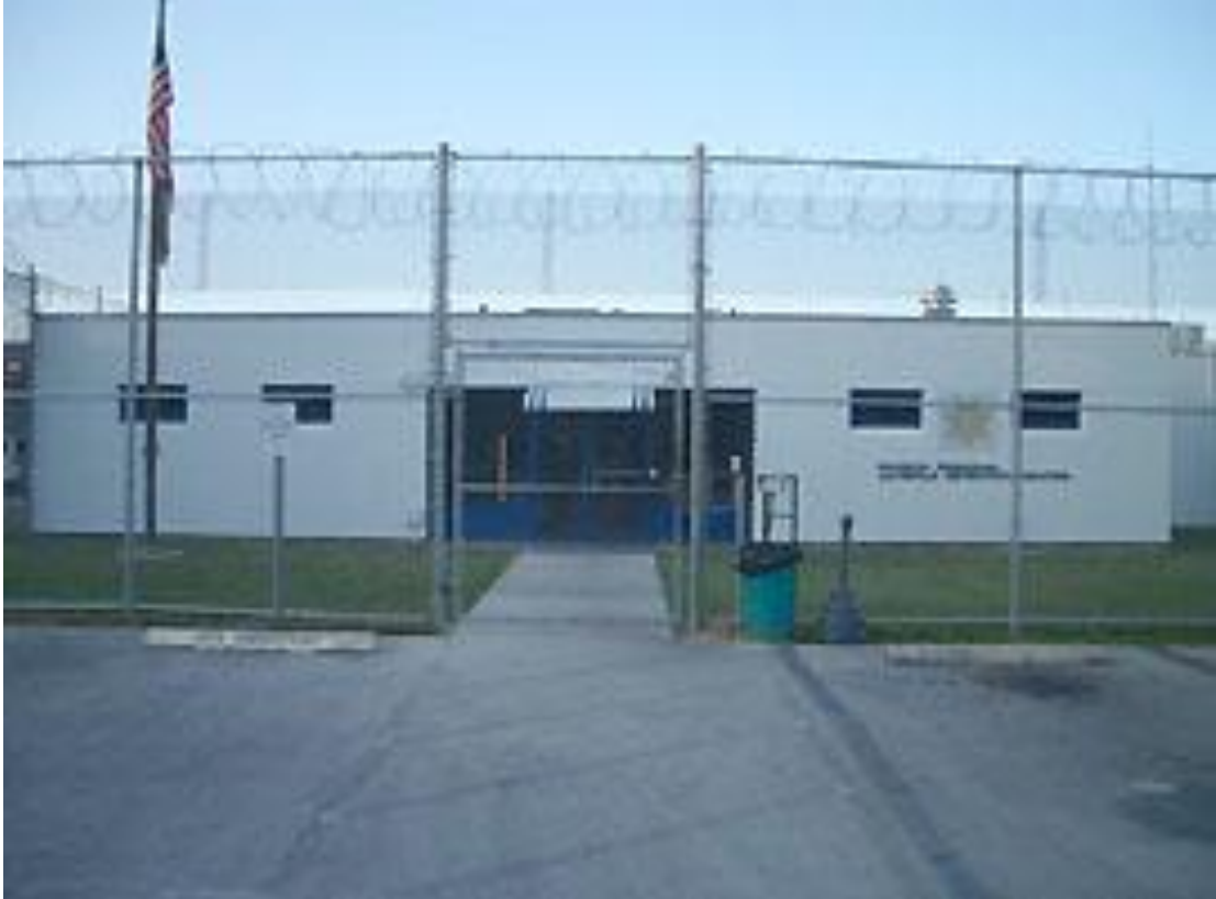
Photo 6. Juvenile Detention Center Campus
