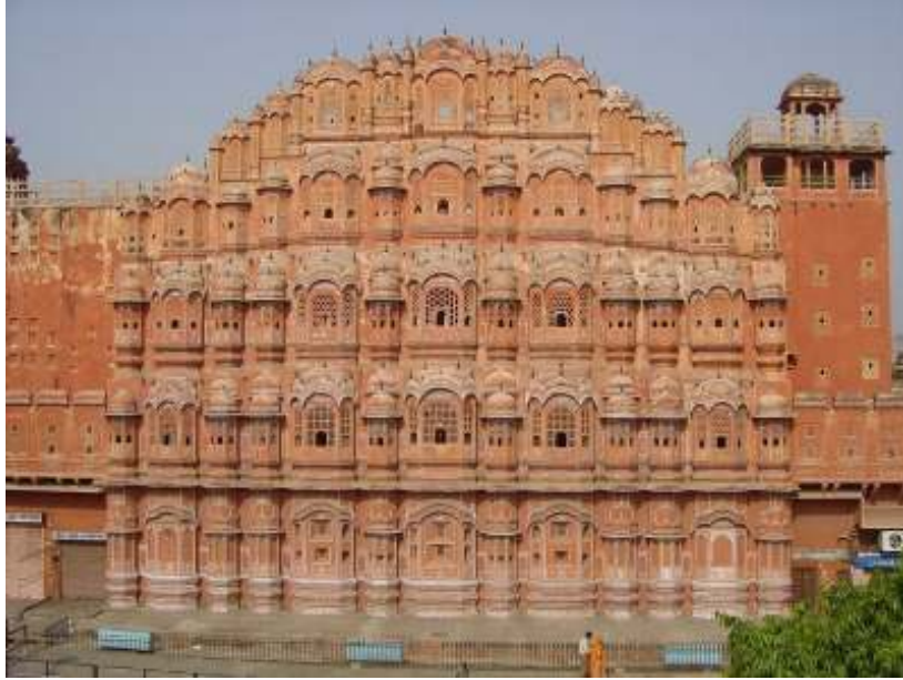
Figure 1.1 – Hawa Mahal (Palace of the Breeze), Rajasthan India where venturi cooling (a passive cooling design) is used. Image courtesy Rajasthan Tourism ( http://www.rajasthantourism.gov.in/ )
