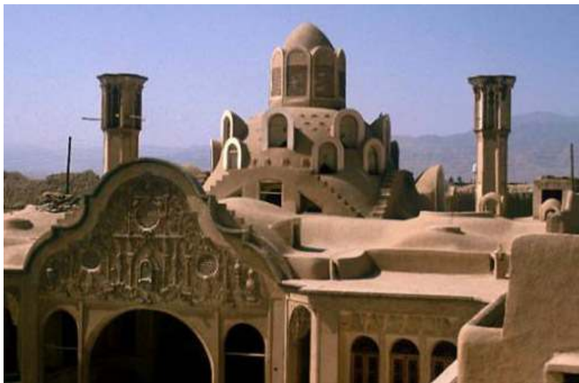
Figure 1.2 – Ancient Persian Architecture with tall wind catchers to cool the interior spaces of the, Borujerdi ha House, in central Iran. Image courtesy Wikipedia.
