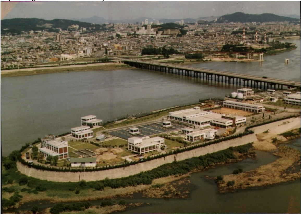
Figure 11. Seonyu Waster Supply Facility in 1980s (Source: http://blog.naver.com/esilvia )
