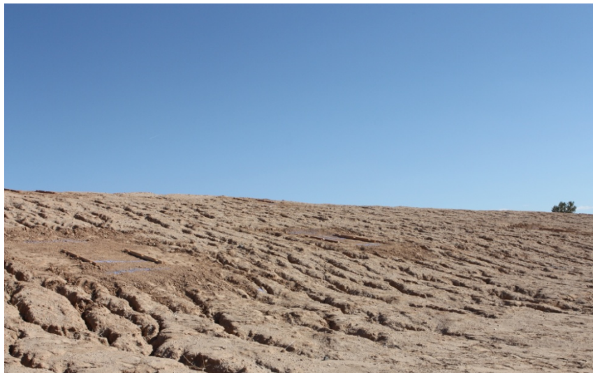
Figure A6: The Slope after Installing the Test Sections
