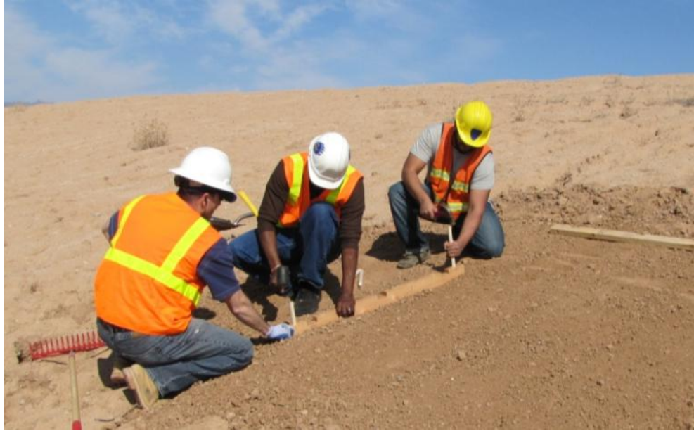
Figure 45: Setting Up the Testing Section
