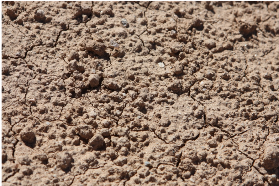
Figure A4: Ground Swelling After Heavy Rain Event
