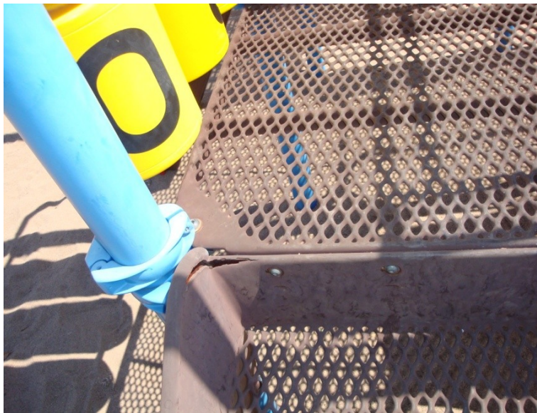
Figure 3: Rusted joint near bridge on playset
