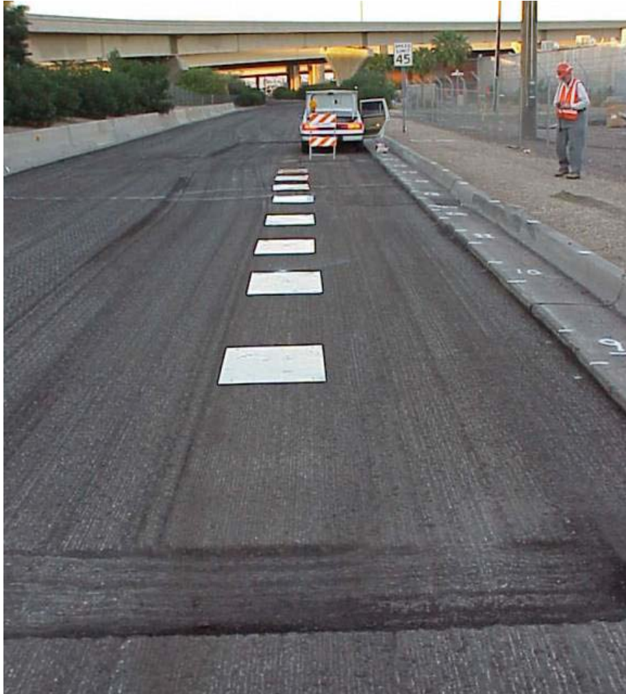
FIGURE 6: Placement of Aluminum Plates Prior to ARAC Overlay
