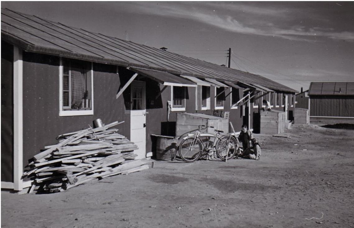
Figure 2.11. Exterior of residential barrack showing initial construction. Window and door awnings are an early alteration made by incarcerated. Pile of lumber was used to both modify accommodations and construct furnishings. Image courtesy of the Amache Preservation Society, McClelland Collection.
