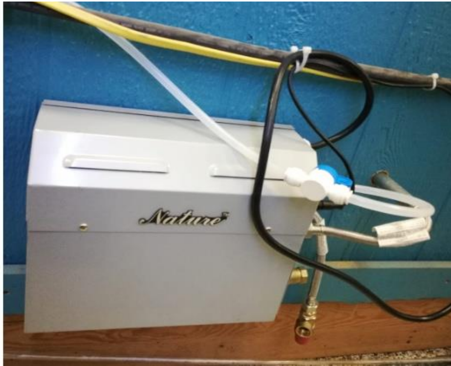
Figure 3.7: Steam generator for humidity delivery
