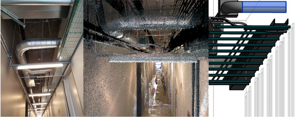
Figure 17: Photograph of the built environment (left), laser scan (center), and resultant model (right)
