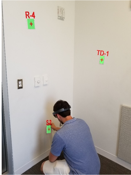
Figure 21: Participant Laying out Electrical Devices with the Virtual Points Shown on the Walls Around Him
