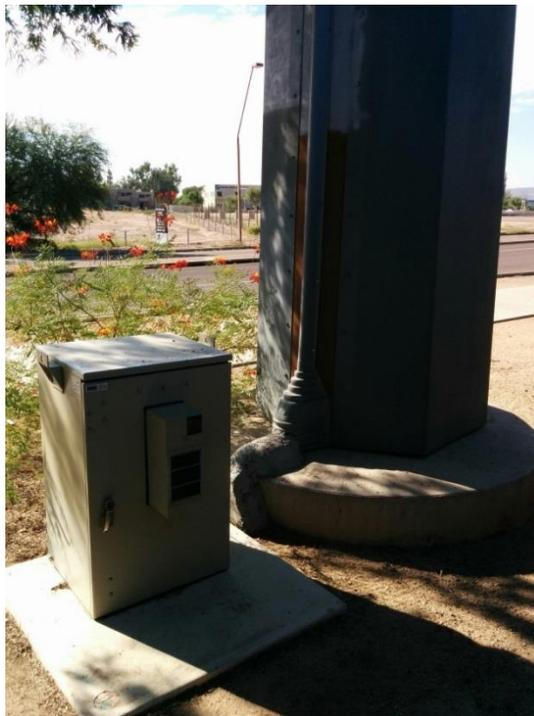
Figure 6.1: DTS Enclosure Installed Next to Riser Pole 24
