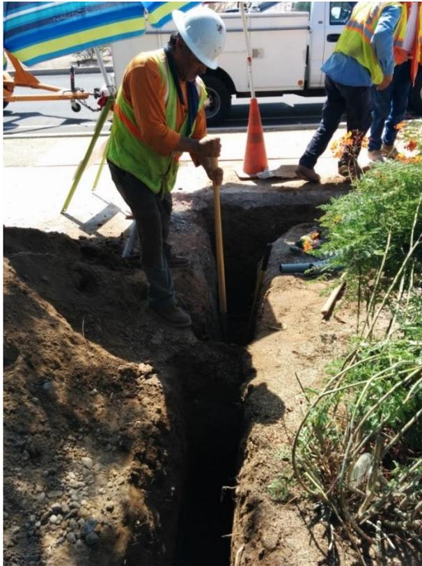
Figure 6.3: Conduit Trench for AC Power Cable to DTS
