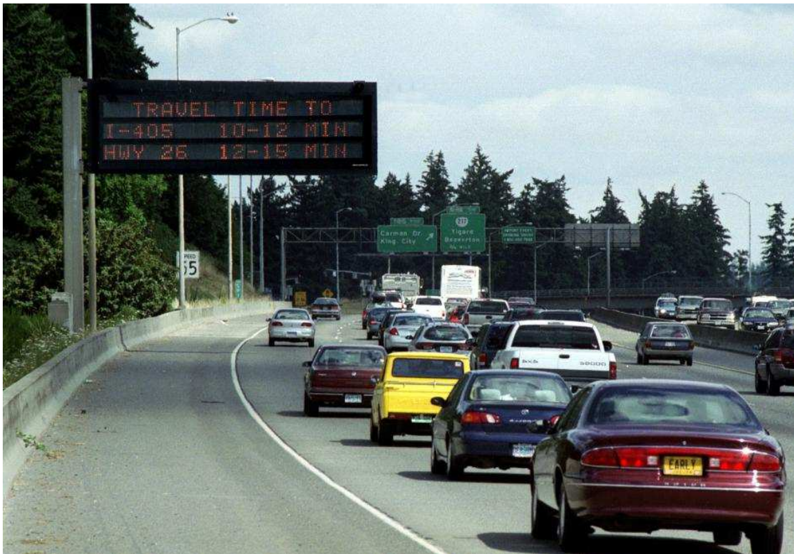
An example of a dynamic message sign time window in Oregon.
