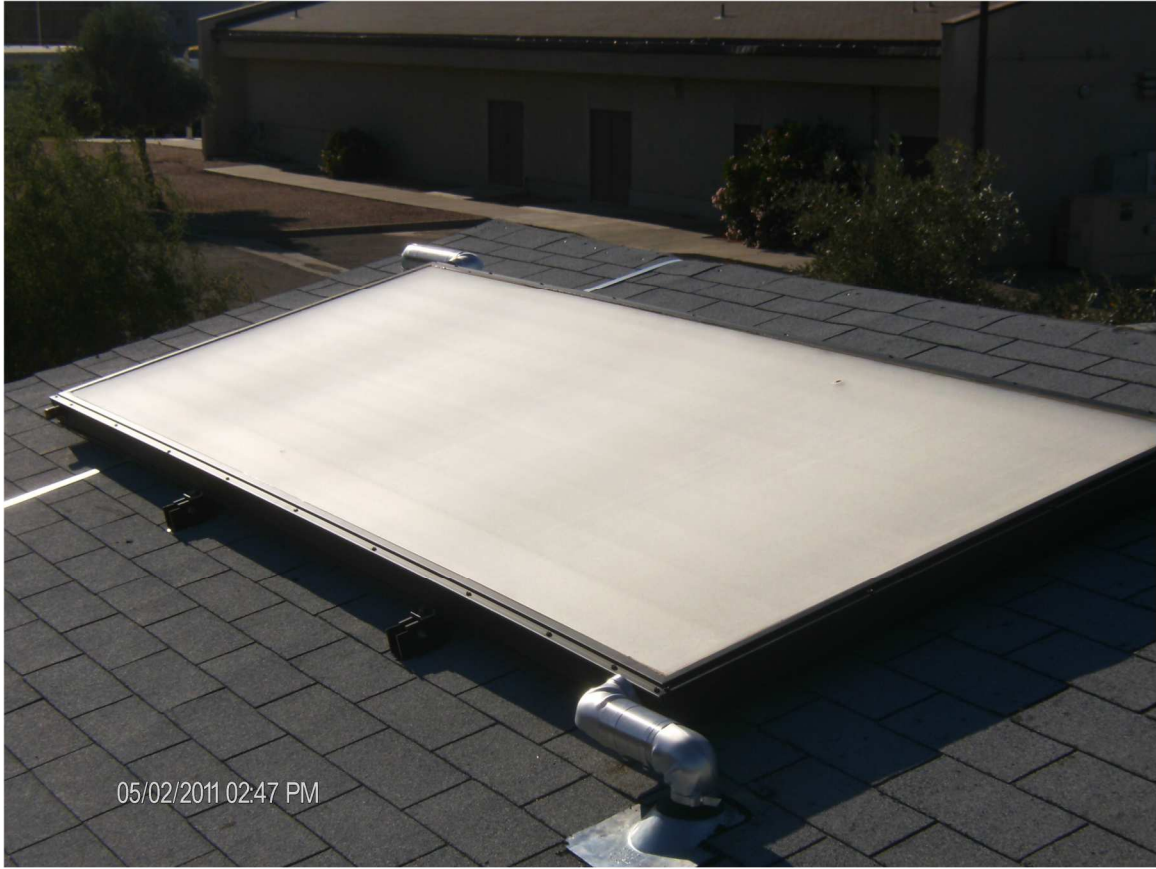
Figure 3.4: Sunearth Flat-plate collector
