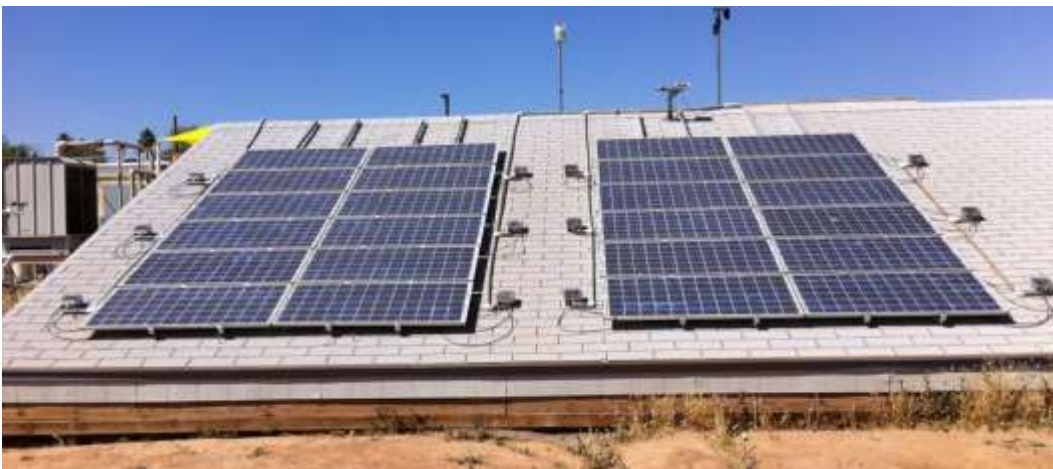
Figure 3.1 The mock rooftop used in the project
