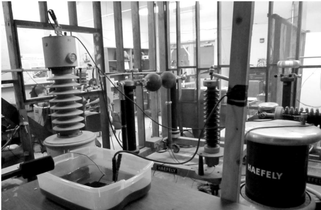
Figure 3.2 The Test Setup for AC Voltage Withstand Test
