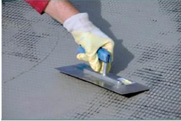
Figure 1.7 Hand lay-up
